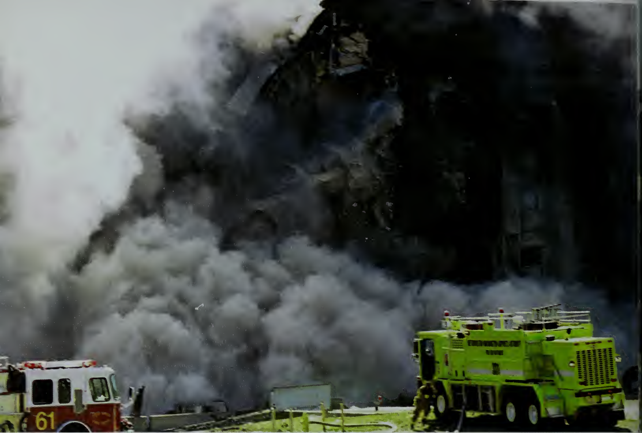
Above: Firefighters pull back as part of the E Ring collapses.
